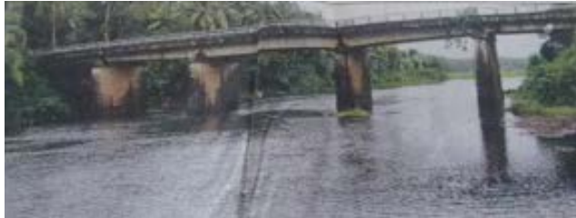
Manjaly river, after the completion of the restoration work through MGNREGS
