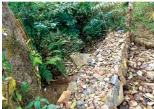
Stone bunding work done through MGNREGS to regulate the flow of a stream in Arunamala colony, Meppadi Panchayat, Wayanad District
