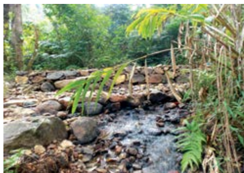
Stone bunding work done through MGNREGS to regulate the flow of a stream in Arunamala colony, Meppadi Panchayat, Wayanad District
