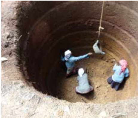
MGNREGS workers digging a well in Varavoor Gram Panchayat, Thrissur District
