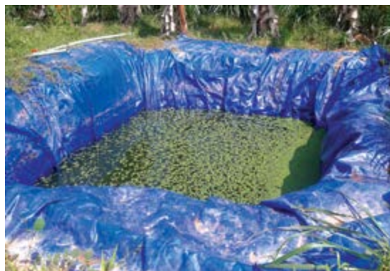
A pond constructed for fish farming in Lalam Block, Kottayam District
