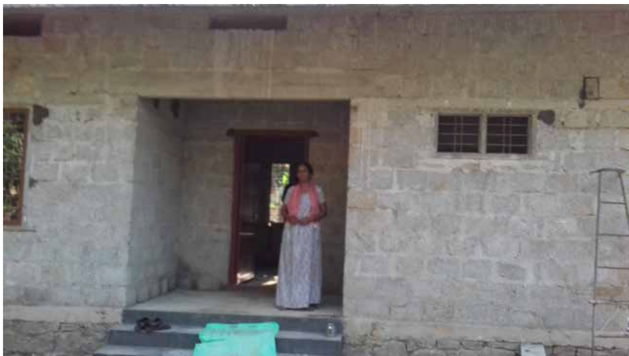
HOUSE CONSTRUCTION UNDER ASHRAYA
